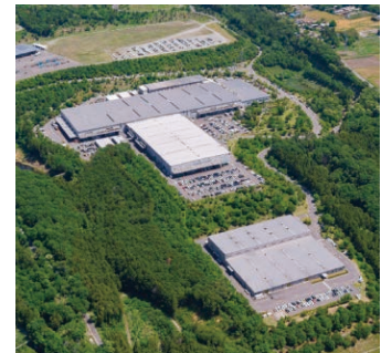
An aerial view of the Sanden Forest/Akagi Plant
