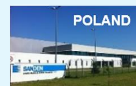
Manufacturing Centre Warehouse
